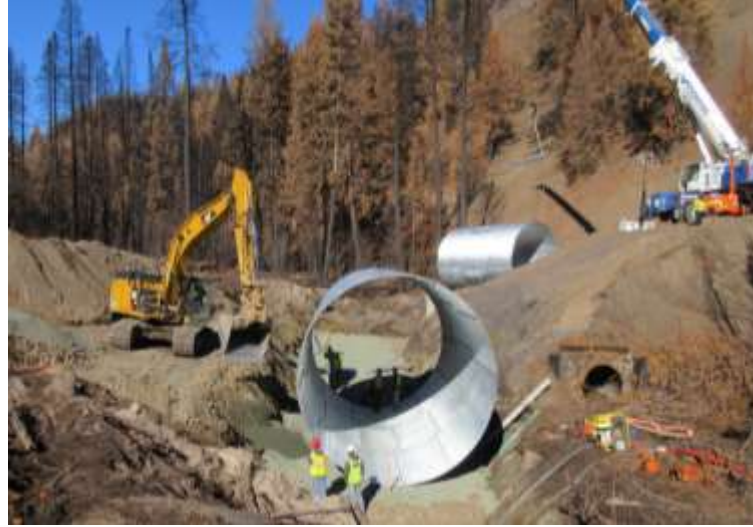
US 395 – Vance and Sheep Creek culvert replacements
